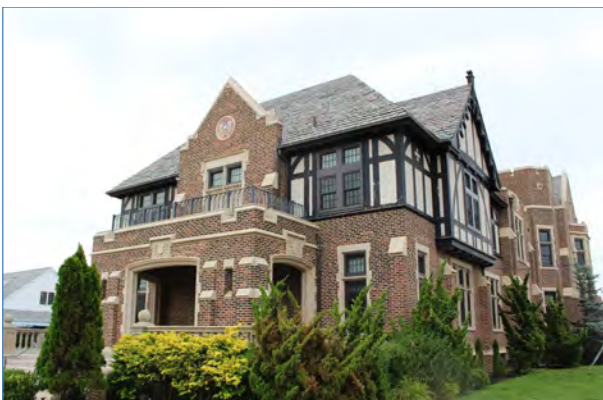
Ventnor City Hall is one of the sites receiving funding from the Sandy Disaster Relief Grants for Historic Properties. p. 16
